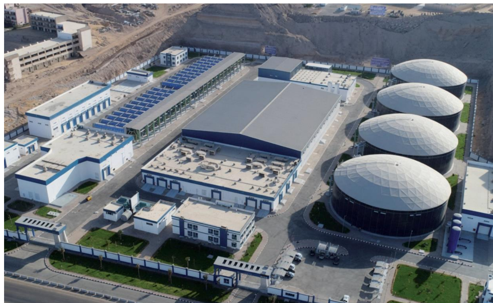
Al Galala SWRO Desalination Plant – aerial view: Main treatment facilities against challenging mountainous terrain with steep elevation differences, managed through earthworks, retaining structures, and coordinated hydraulic and structural design. © ECG; Dorsch Global
