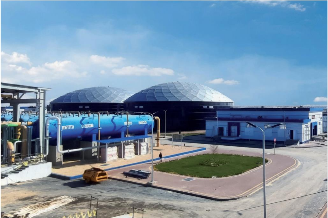
Al Arish SWRO Desalination Plant – Commissioning: Completed commissioning-stage facility showing successful design implementation and integration of major treatment units. © ECG; Dorsch Global
